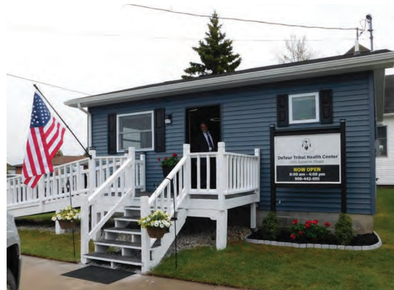
Sault Tribe's DeTour Health Center opened on on May 19.
